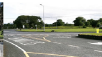
Road Realignment and Landscaping at Bohola
